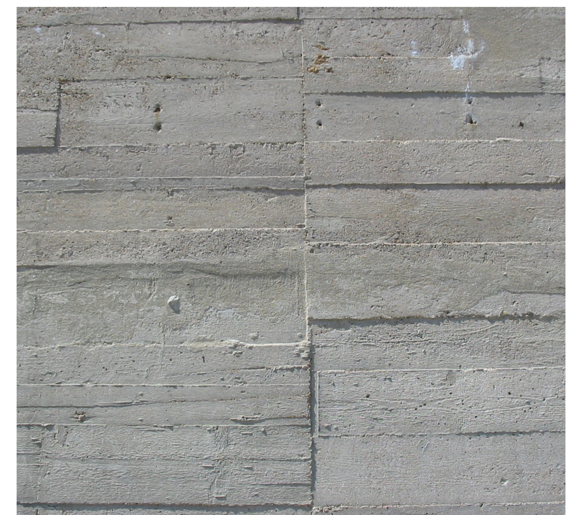
Board Formed Concrete Creates a neutral shell to the vibrant liner of the parklet contrasting in it's texture and mimics a more organic exterior .
